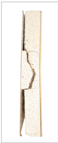
Rigid plastic wall panel - complete structural failure.
