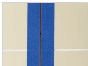
After adhesive dries one hour, remove nail and protect face with tape.
