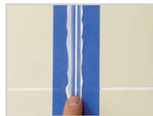
Using your finger, place a slight indentation in the gap.
